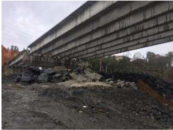
Photo 3 Concrete spillage at Site
